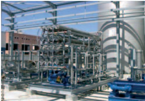
distributed in a series of independent loops (each one composed by recirculation pump, instrumentation, membranes) with series/parallel configuration of the membranes
