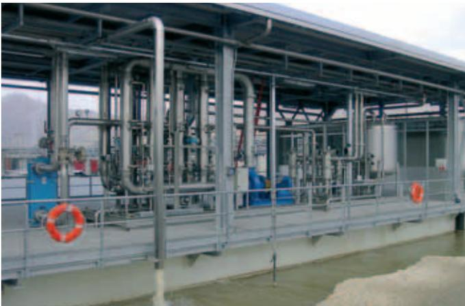
In the oxidation tank biodegradable substances are eliminated and ammonia and nitrogen-based compounds can also be removed, while the membrane filtration system removes 100% of the suspended solids giving a fully sterilized treated water. One of the advantages of bioHAR® system is the stable filtration rate without membrane cleaning problems.
